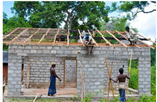
Housing construction taking place with integration of building guidelines
